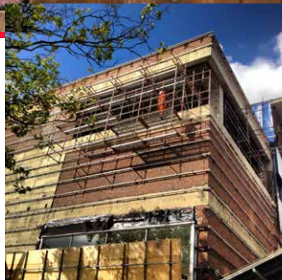
Project in de steigers
